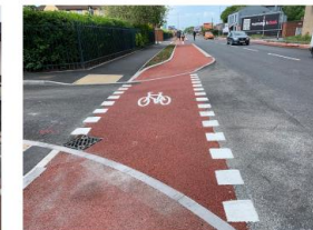
Priority to cyclists can be provided at side roads even in industrial areas using coloured bollards and markings.
